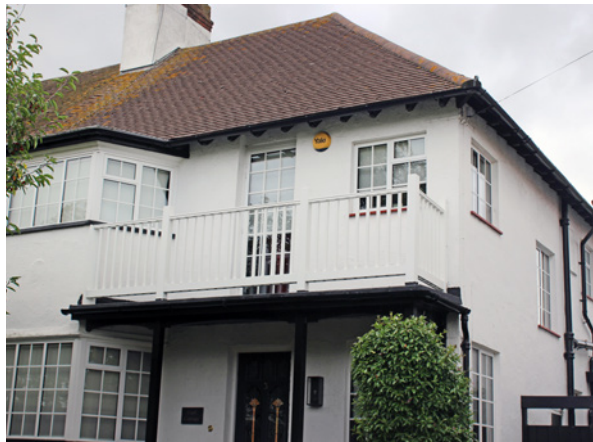
A modern balcony extension
