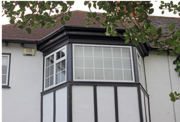
Unsympathetic window units
