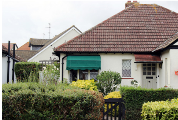
Replacement concrete tiles and a Dutch canopy added to a window
