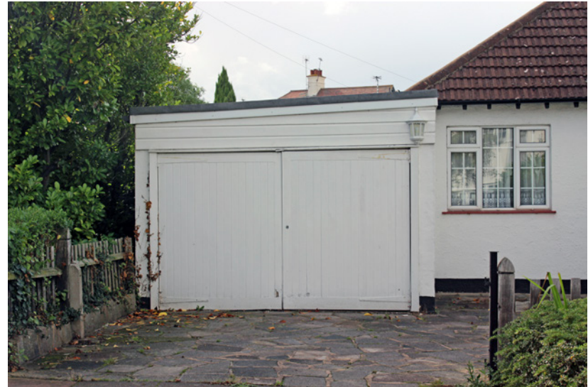
Flat-roofed garage extension
