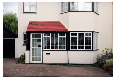
Example of an inappropriately infilled porch
