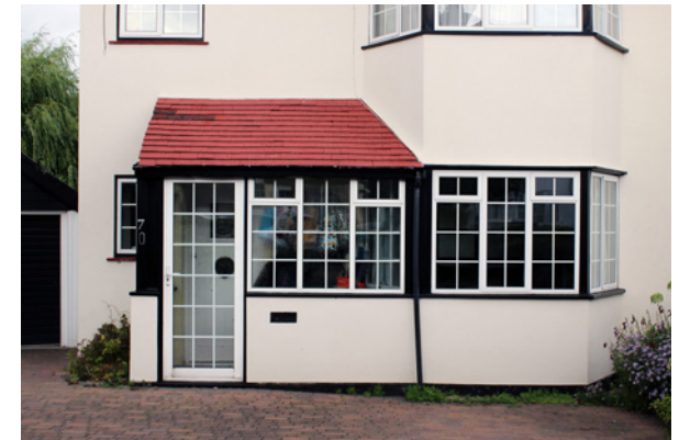
Example of modern porch infilling the space next to a bay window
